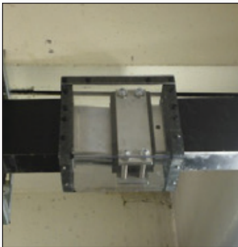
ITEC.BAR™ GPA range: conductors in aluminium E-AlMgSi
